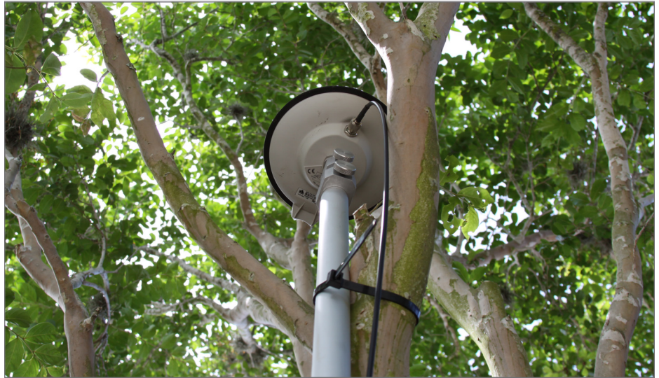
Figure 13 Typical Canopy Environment
